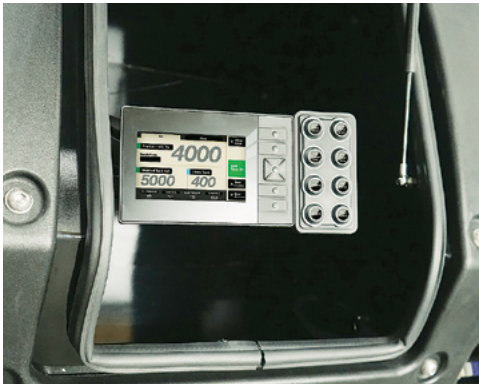
The external G-Hub Controller located in the storage box of the Quick Filling Station.
